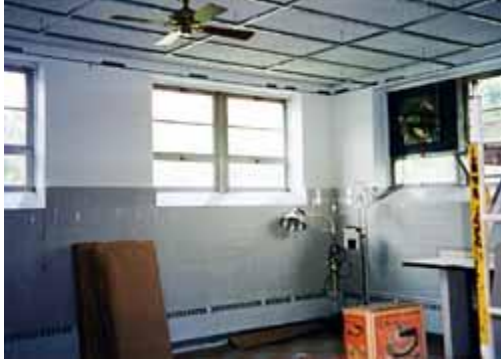
Renovation of Room 15
